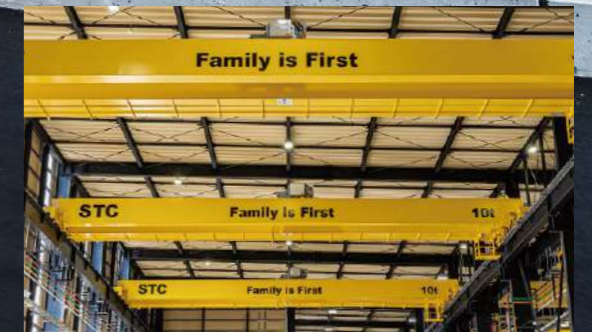
Crane embossed with the "Family is First" slogan in the factory building
