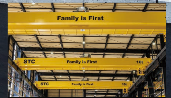
Crane embossed with the "Family is First" slogan in the factory building
